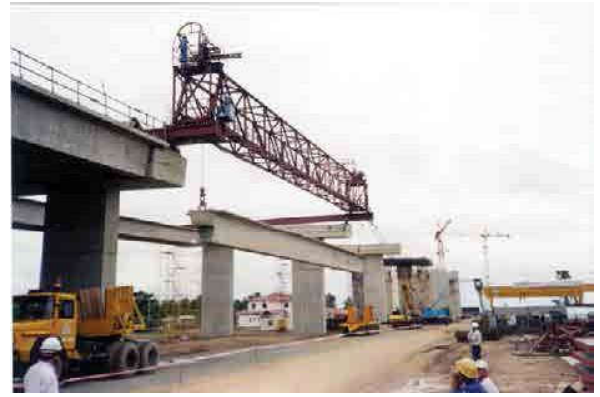
Dàn lao phóng dầm / Lifting Truss Quatity: 02 sets Capacity: 80 tons
