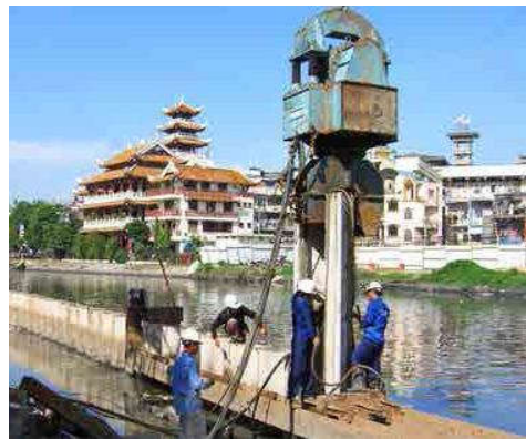
Búa rung / Vibro Hammer Quatity: 05 units Capacity: 40 - 90 KVA
